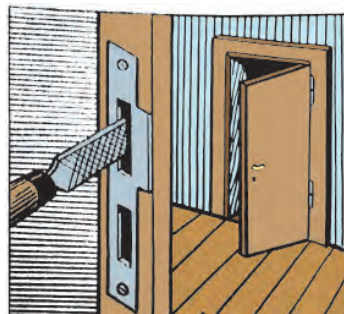
85-rasm. Uyalarni egovlab moslash.
